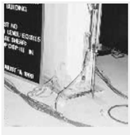
a) Negligible observed damage at the wall base
